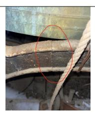
This is an example of a head bolt that deteriorated over time, but cannot be seen through the bell support beam.
