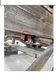
Cast iron bell stands have a tendency to crack over time. This is very dangerous and requires immediate attention.
