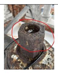
Vibration over time, along with old, dried and shrinking timbers, will loosen and spin off nuts, resulting in bell structure failure.
